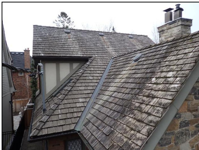
Shingles are in good overall condition
