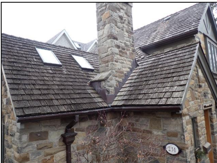
Shingles are in good overall condition
