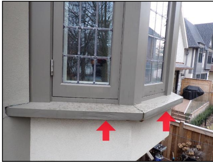
Rot suspected at window sill
