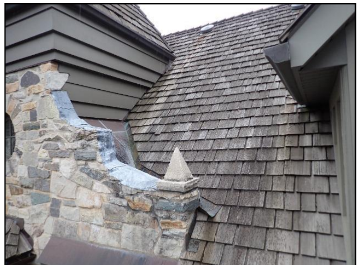
Shingles are in good overall condition
